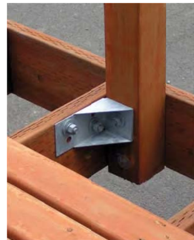
FIGURE 2—TYPICAL BRACKET INSTALLATION
