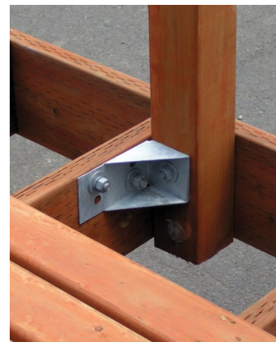
FIGURE 2—TYPICAL BRACKET INSTALLATION
